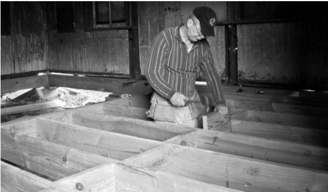
Local Historian, Bernie Rudberg, restoring the floor of the Hopewell Junction Railroad Depot.
